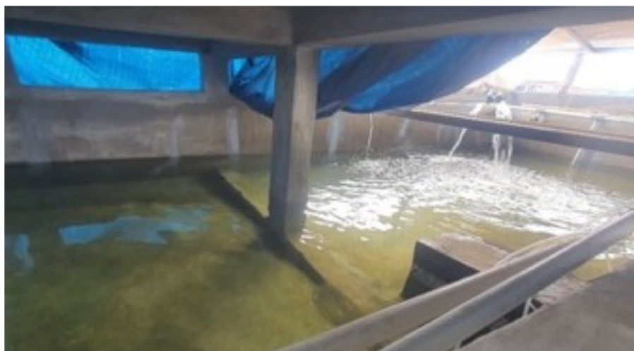
Figure 3. Test Pond with RAS filtration system (Recirculating Aquaculture System)
