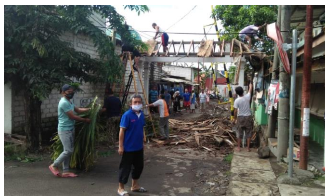
Figure 3. Gotong Royong to Build a Gate
